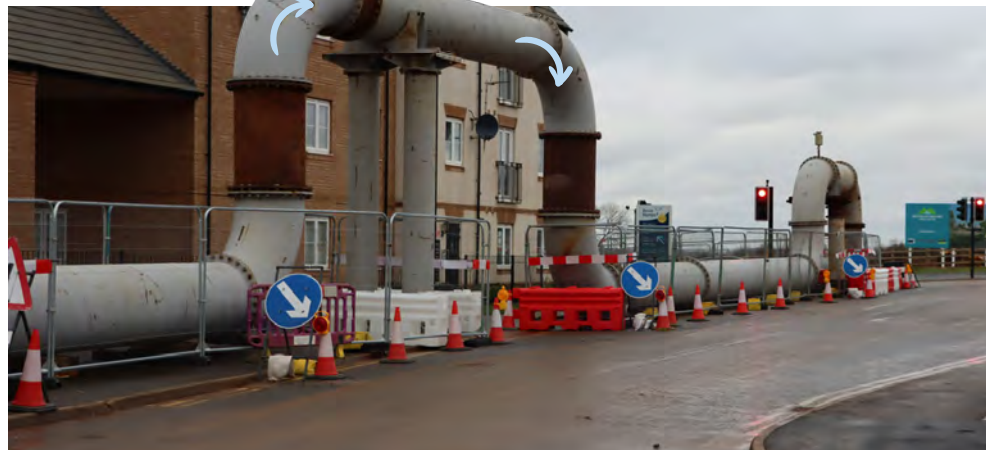
Overground sewer constructed in nine days to avoid pollution in Wellingborough.
